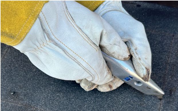
Remsa 25 x 500 mm skärs i underlaget.
